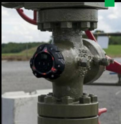
Gas detection and local alarms for high-risk areas. Just turn on your ALTAIR io360 Gas Detectors and deploy where needed.
